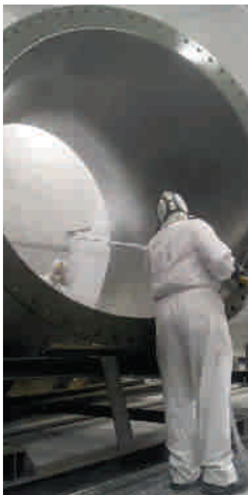
Applying Accoshield corrosion protection coating
