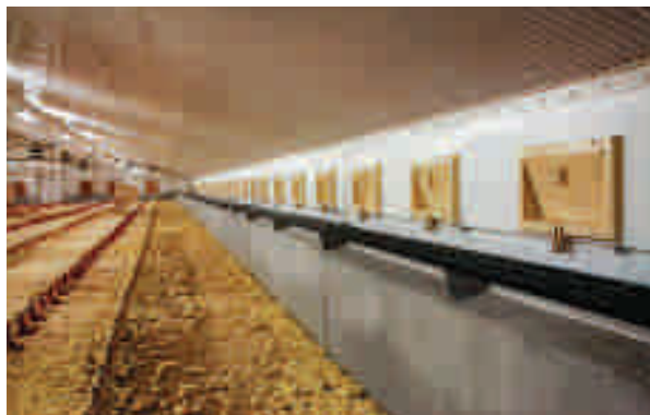
TPI's air inlet valves in a chicken barn
