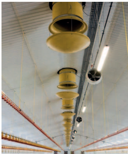
TPI Polytechniek – ventilation in a pig house
