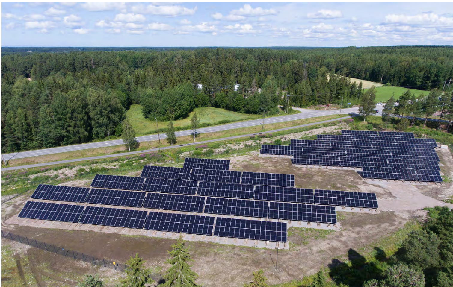
Solar park at Coreplast Laitila Oy.
