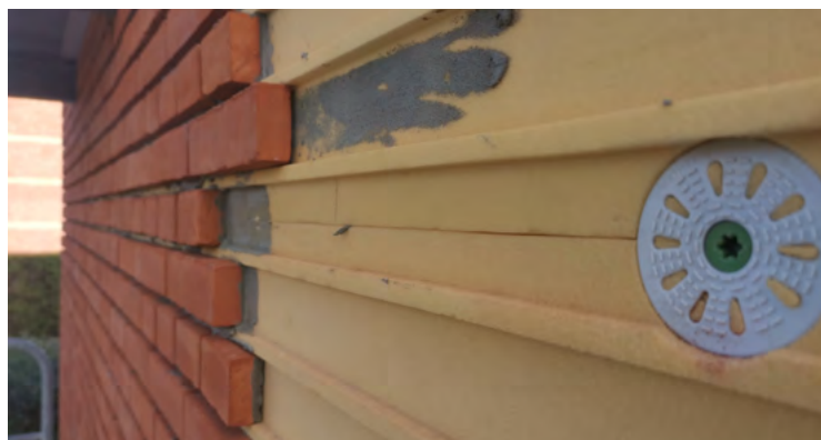
Tinby Skumplast supplies insulation sheets to Briiso for their façade insulation system.
