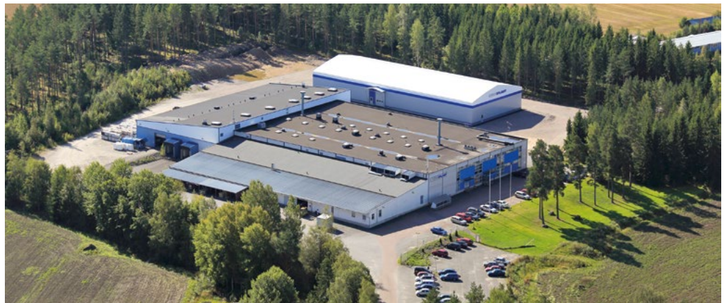
Coreplast's injection-moulding factory in Laitila, Finland.
