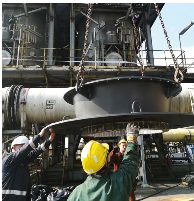
Corrosion protecting Accoshield® coating – part for the chemical industry
